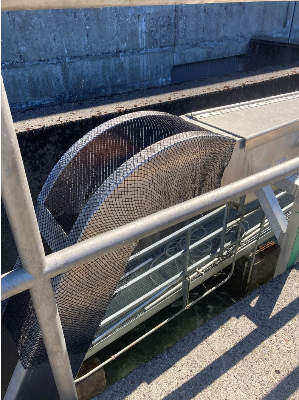
Photo 2: Netting was added to the flume portion of the AFF trap, adjacent to walkway.
